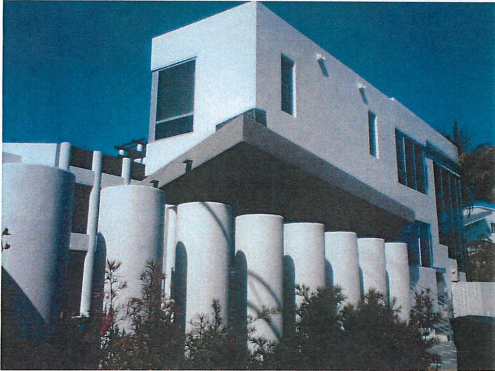
SIDE VIEW -- PHOTOS TAKEN ON 03-31-2012
