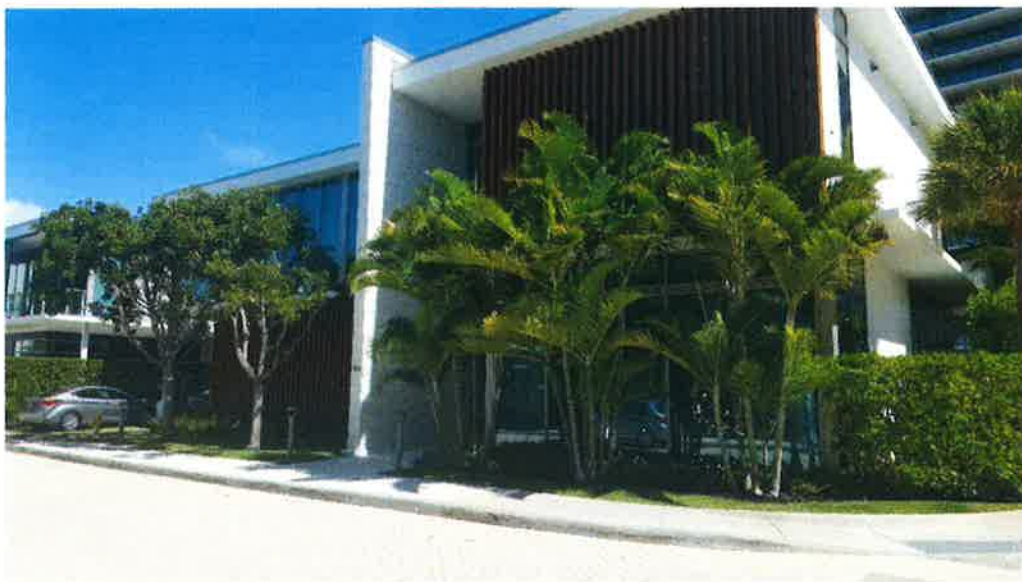
VILLA 1 – WEST LOOKING NORTHEAST 2-20-2019
