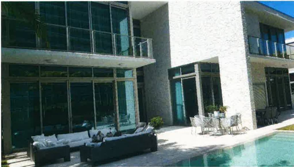
VILLA 1 – EAST LOOKING NORTHWEST 2-20-2019
