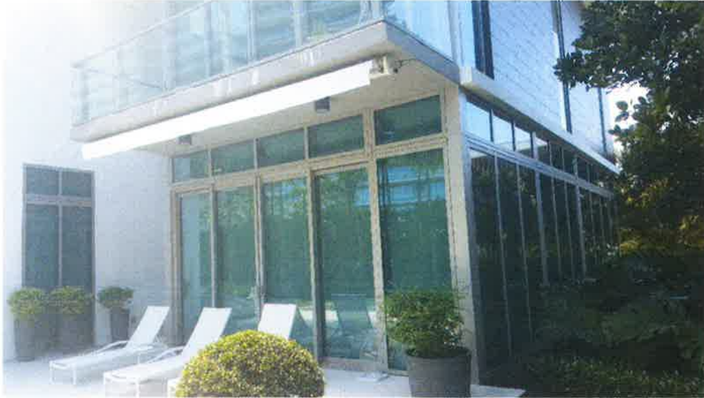
VILLA 2 – NORTHEAST CORNER LOOKING WEST 2-20-2019
