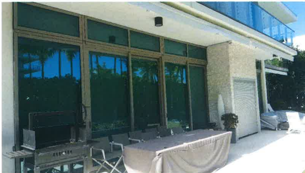
VILLA 2 – EAST SIDE LOOKING NORTH 2-20-2019
