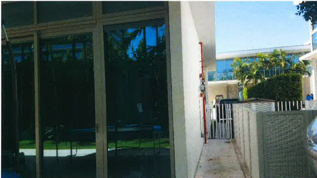
VILLA 3 – NORTH SIDE LOOKING WEST 2-20-2019
