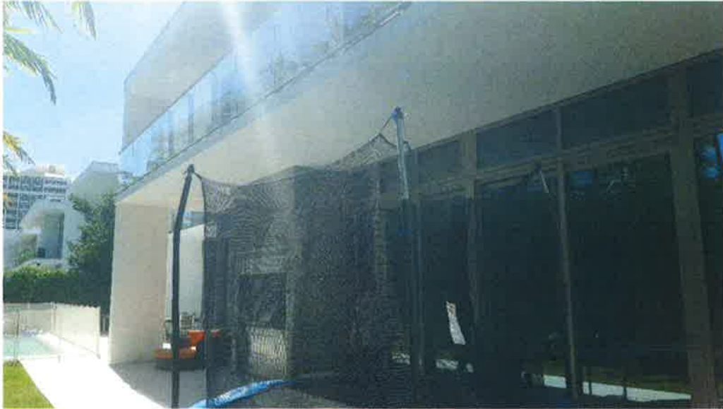
VILLA 3 – EAST SIDE LOOKING SOUTH 2-20-2019
