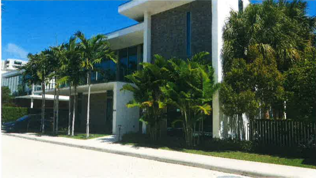
VILLA 3 – WEST SIDE LOOKING NORTHEAST 2-20-2019
