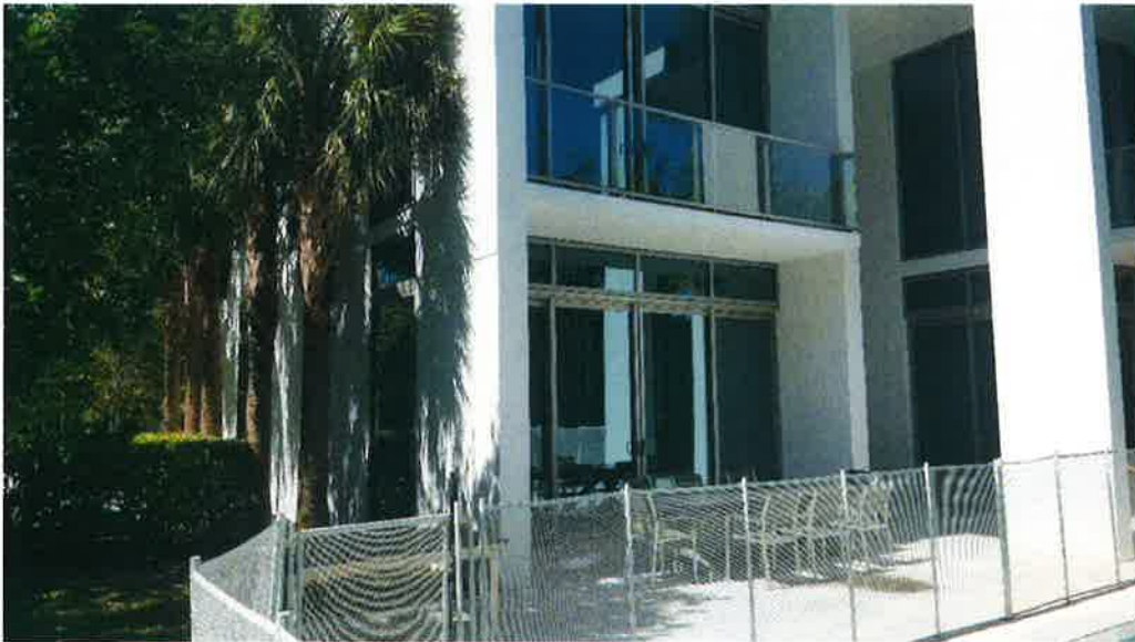
VILLA 3 – SOUTHEAST CORNER LOOKING WEST 2-20-2019
