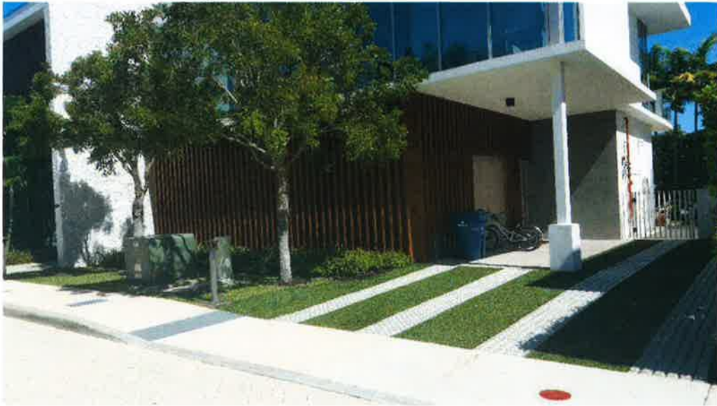
VILLA 4 – SOUTHWEST CORNER LOOKING EAST 2-20-2019
