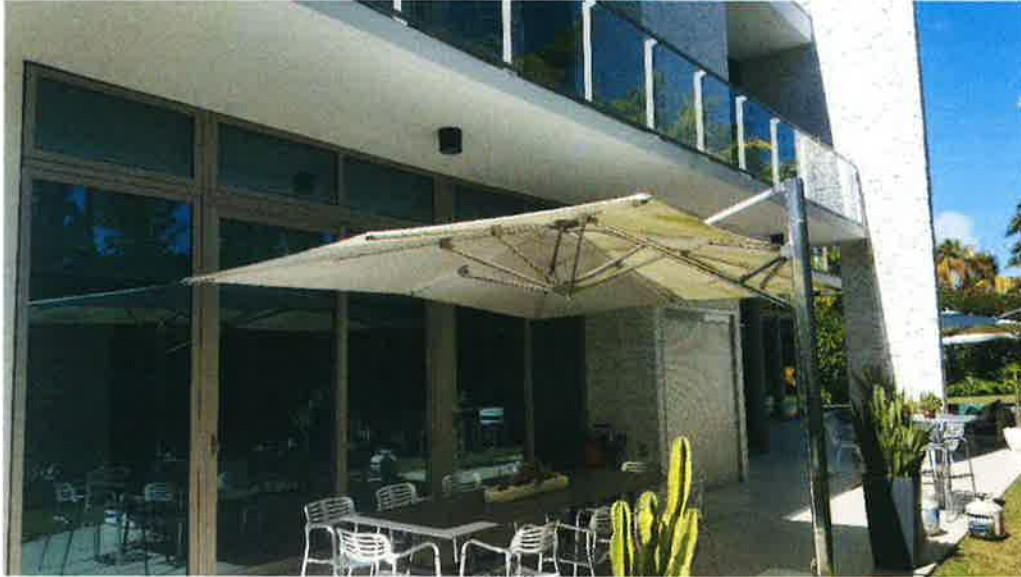
VILLA 4 – EAST SIDE LOOKING NORTH 2-20-2019
