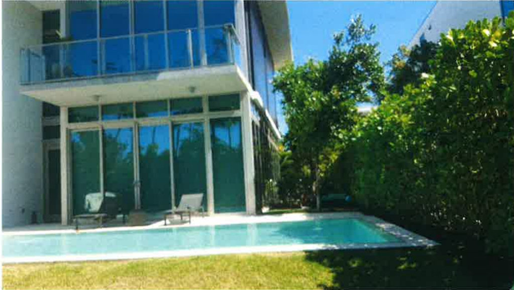
VILLA 5 – SOUTHWEST CORNER LOOKING EAST 2-20-2019
