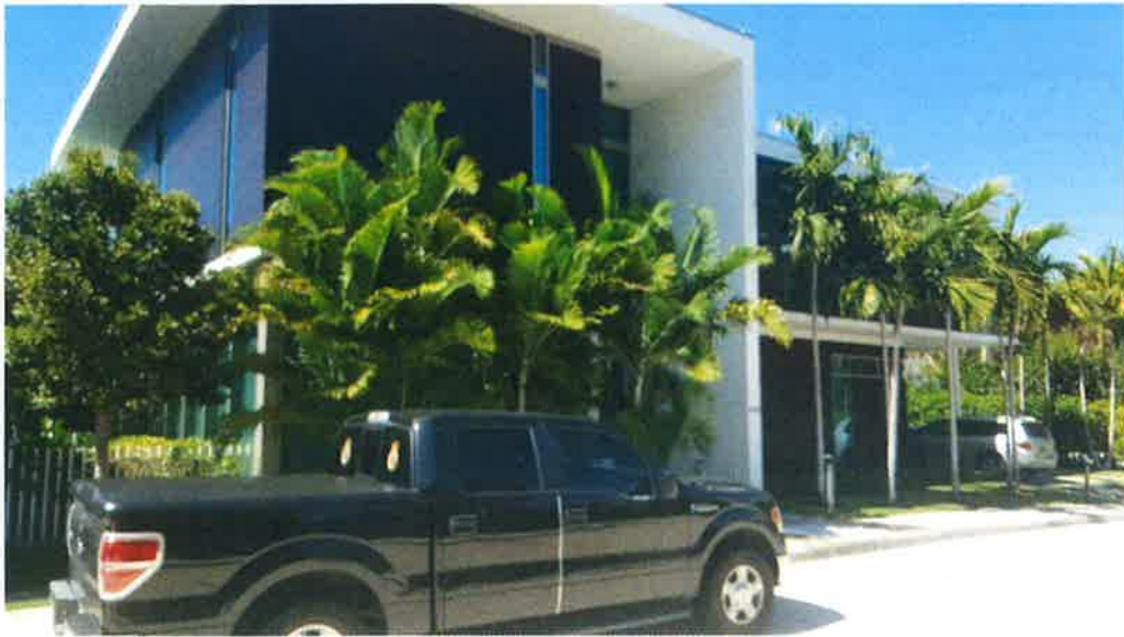
VILLA 5 – EAST SIDE LOOKING NORTHWEST 2-20-2019
