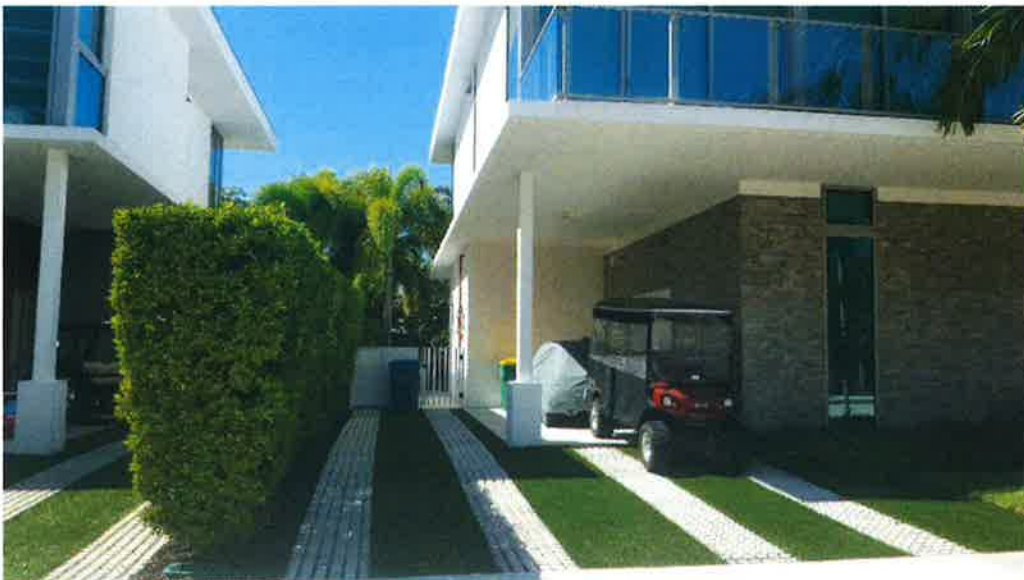
VILLA 6 – SOUTHEAST CORNER LOOKING WEST 2-20-2019
