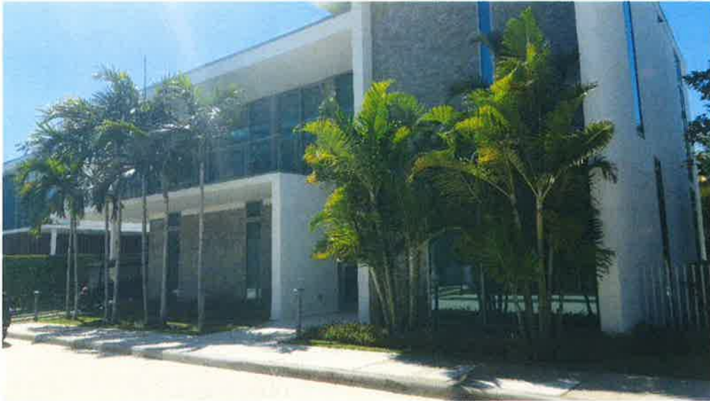
VILLA 6 – EAST SIDE LOOKING SOUTH 2-20-2019
