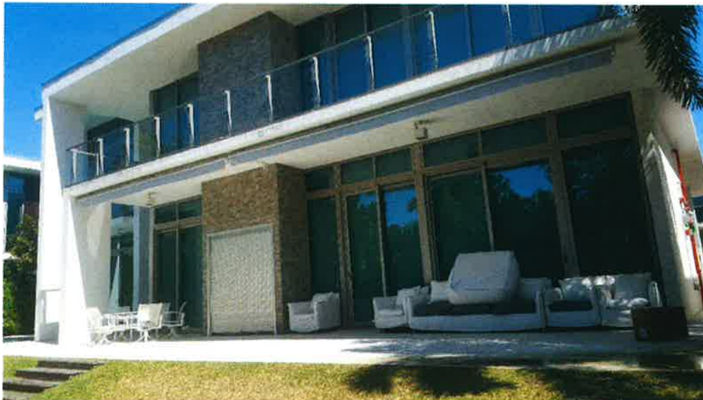
VILLA 6 – WEST SIDE LOOKING NORTH 2-20-2019
