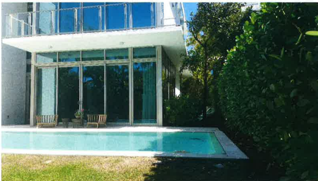
VILLA 7 – SOUTHWEST CORNER LOOKING NORTHEAST 2-20-2019
