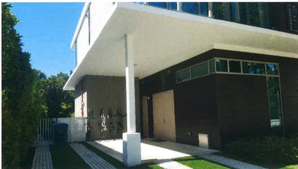
VILLA 8 – SOUTHEAST CORNER LOOKING WEST 2-20-2019
