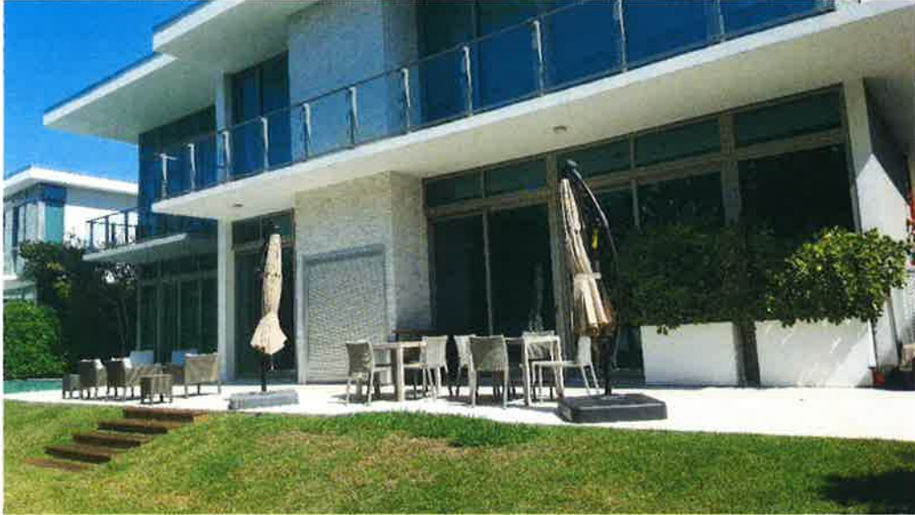
VILLA 8 – WEST SIDE LOOKING NORTH 2-20-2019
