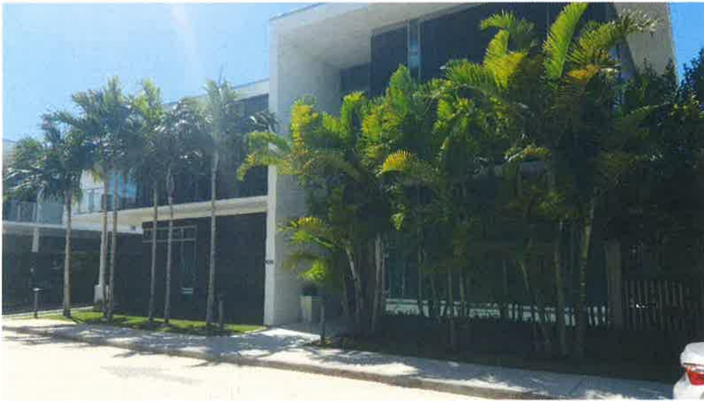
VILLA 8 – EAST SIDE LOOKING SOUTH 2-20-2019
