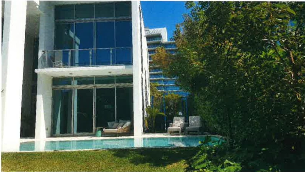
VILLA 9 – SOUTH SIDE LOOKING EAST 2-20-2019
