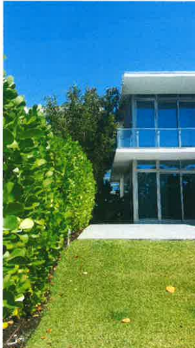
VILLA 10 – SOUTH SIDE LOOKING EAST 2-20-2019
