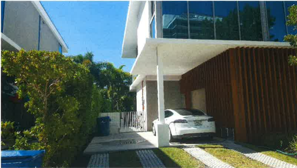
VILLA 10 – SOUTH SIDE LOOKING WEST 2-20-2019
