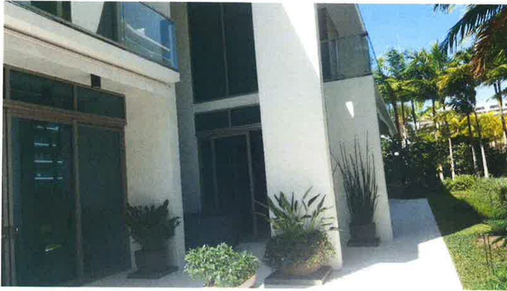
VILLA 12 – EAST SIDE LOOKING SOUTH 2-20-2019
