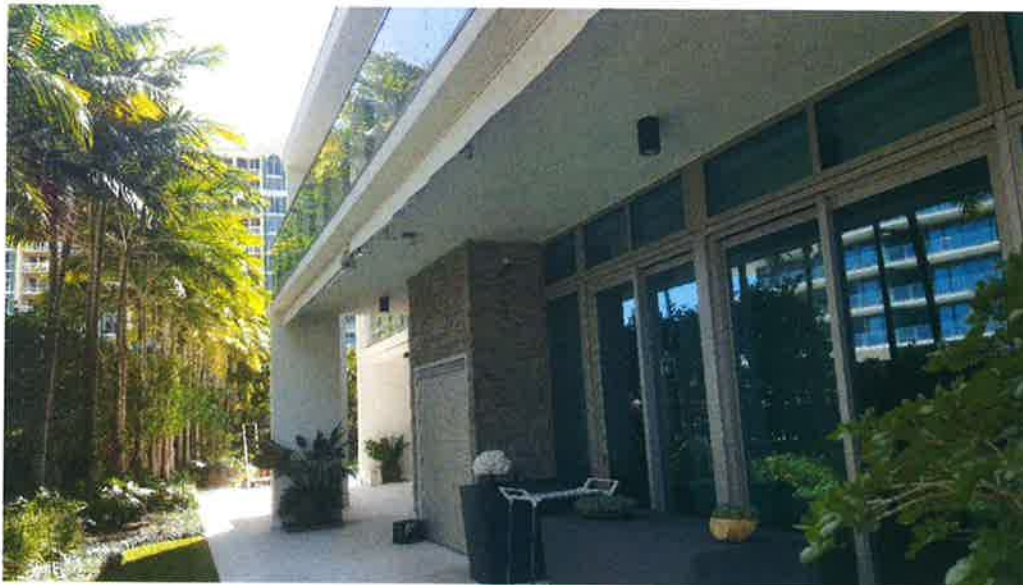
VILLA 12 – EAST SIDE LOOKING NORTH 2-20-2019
