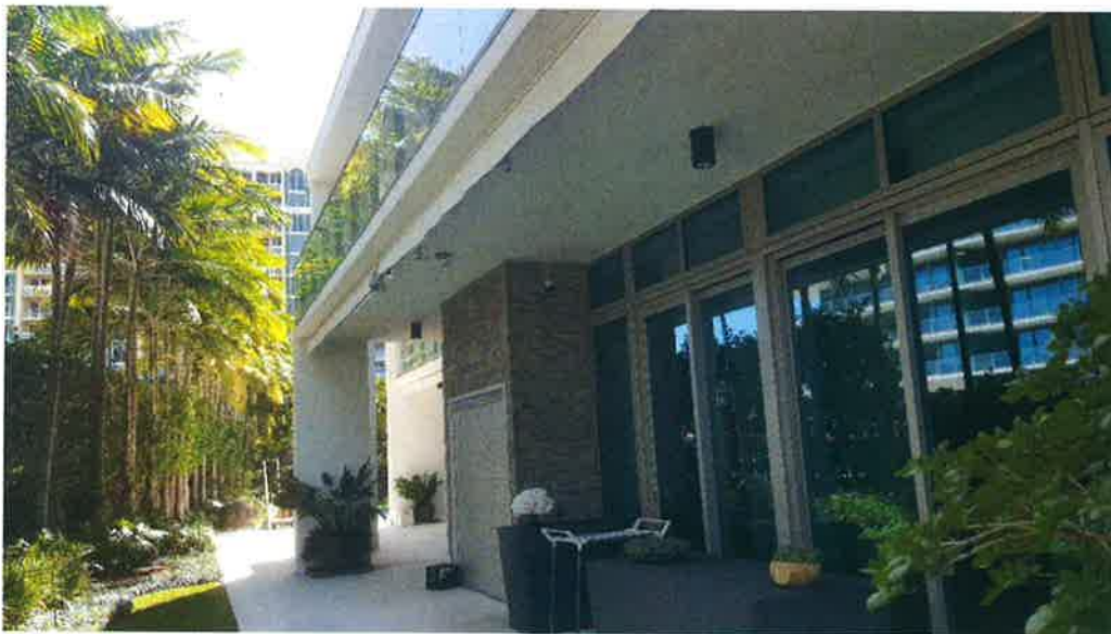
VILLA 12 – EAST SIDE LOOKING NORTH 2-20-2019
