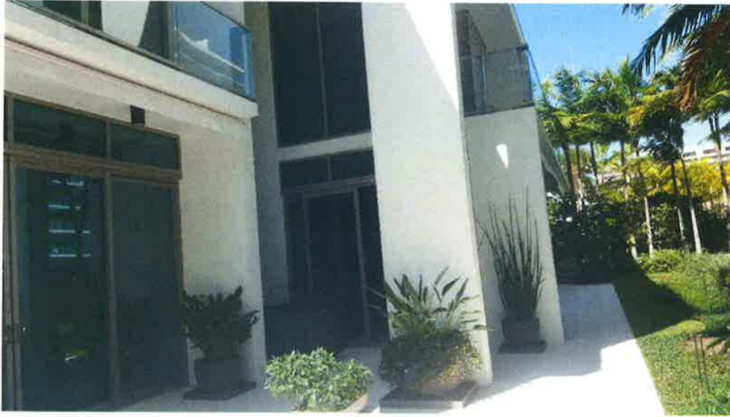
VILLA 12 – EAST SIDE LOOKING SOUTH 2-20-2019
