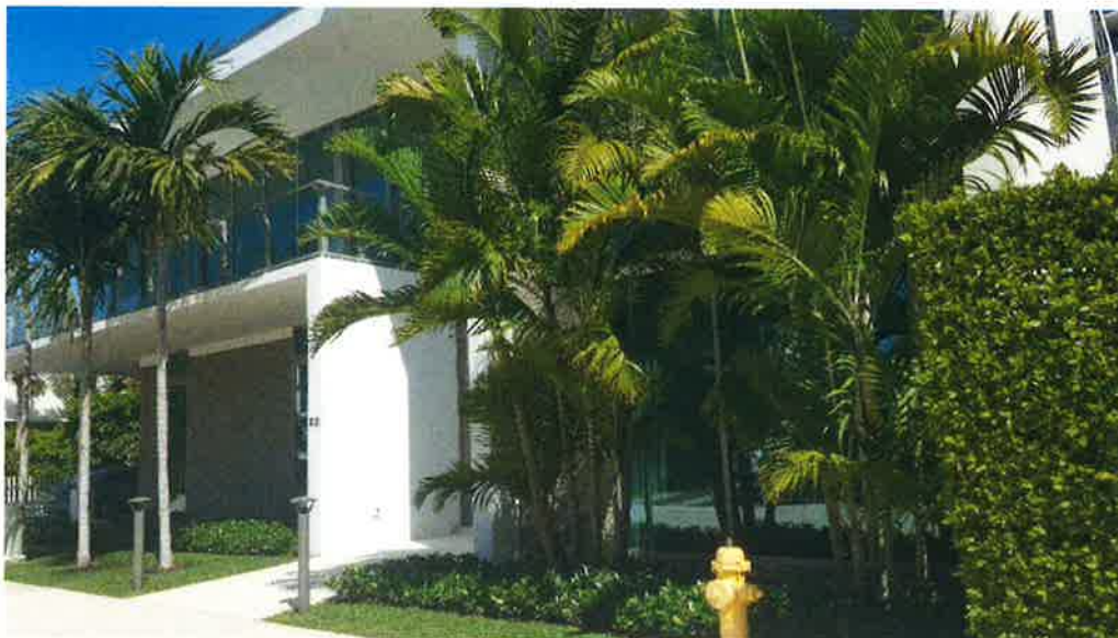
VILLA 12 – WEST SIDE LOOKING NORTH 2-20-2019
