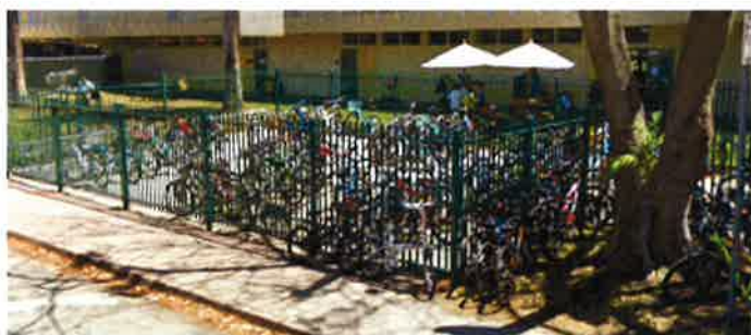
Existing Deficient Bike Parking/Storage
