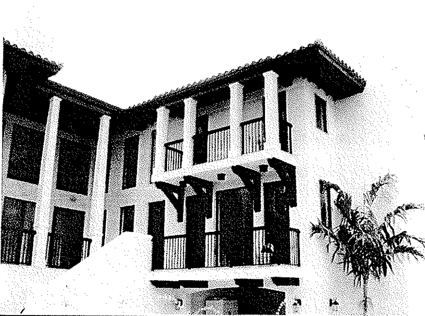
BUILDING REAR VIEW (PICTURE TAKEN ON APRIL 17, 2009)
