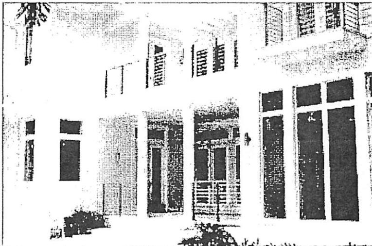
BUILDING REAR VIEW (PICTURE TAKEN MAY 17, 2011)
